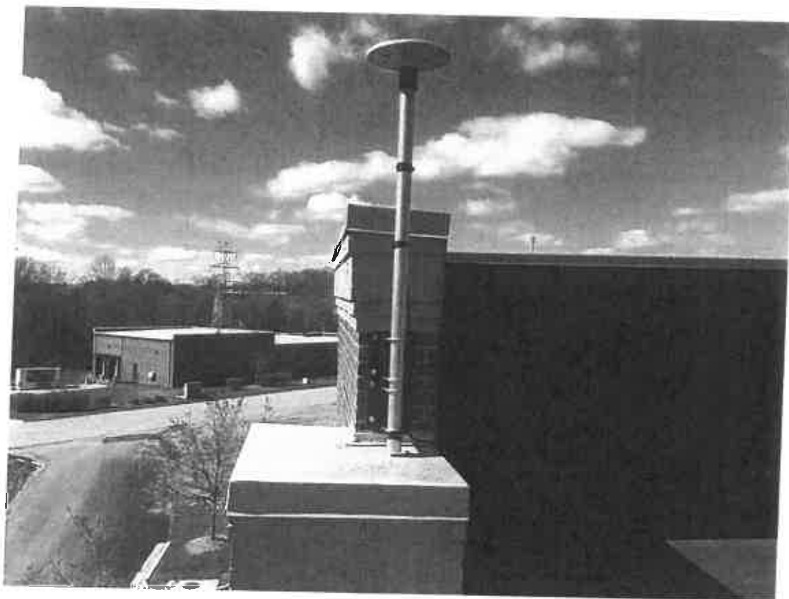
GPS antenna mounted on a brick wall.
